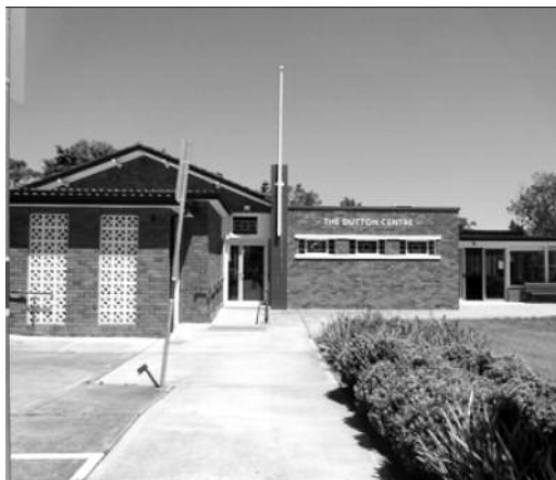
写真資料① Dutton Community Centre
