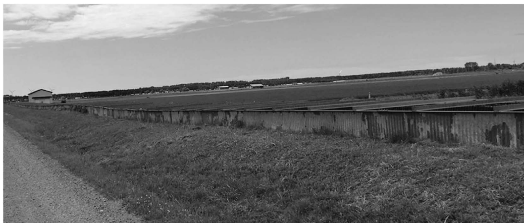
Fig. 1 Differential settlement of channel (Some parts are deformed while others are not so deformed. This phenomenon has accelerated the channel degradation.)
