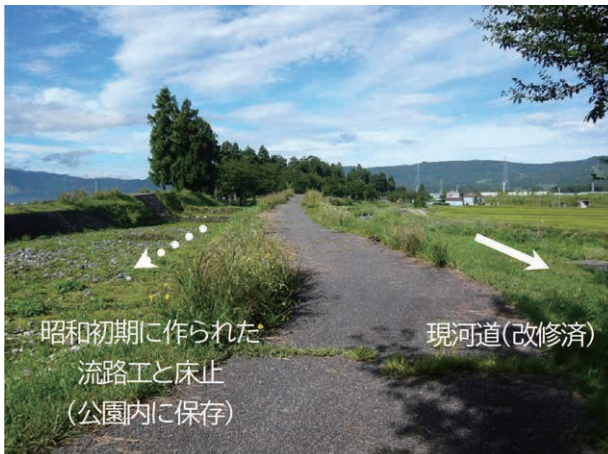
図-9 現在の鎌倉沢川砂防流路工 Fig.9 Current Kamakurasawa River Sabo Channel works
