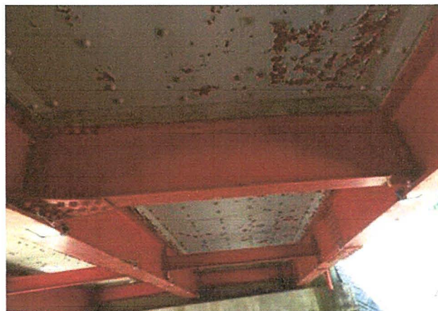
(a) 床版取替前
