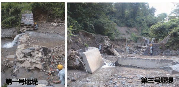
図-7 豪雨による被災状況 (鎌倉沢川) Fig.7 Damage caused by heavy rain (Kamakurasawa River)
